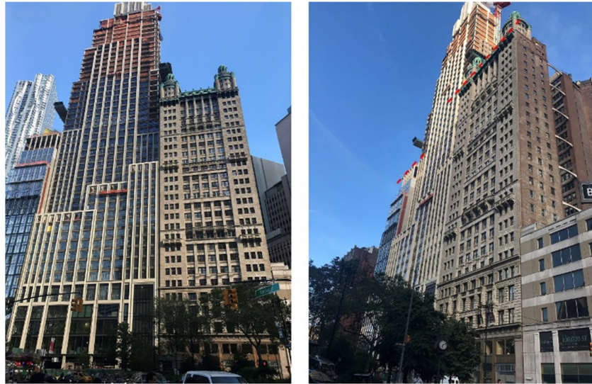
Photographs of the Adjacent Buildings in Progress, July 2019
