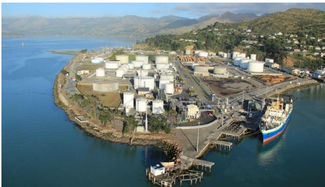
Figure 1: Lyttelton Port showing a vessel moored at the existing Oil Berth
