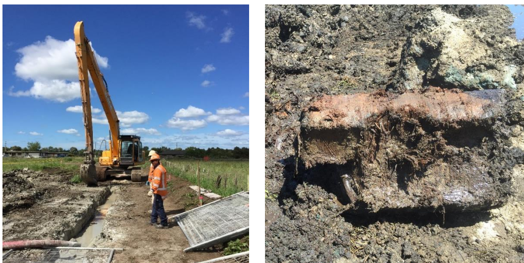
Figure 7: Slurry wall installation and obstruction removal
