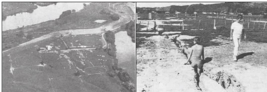
Figure 3: Historical photographs outlining the occurrence of liquefaction in Whakatane following the 1987 Edgecumbe earthquake (Collated from Christensen (1995)).
