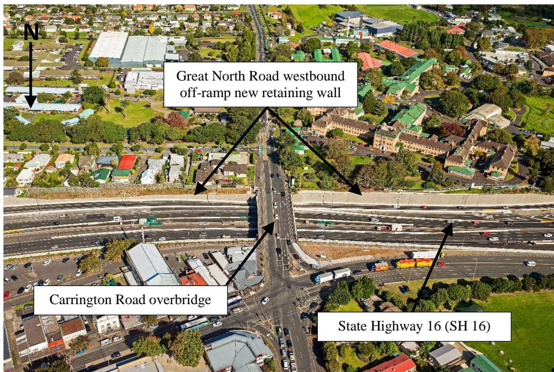
Figure 1: Aerial view of the Great North Road westbound off-ramp new retaining wall
