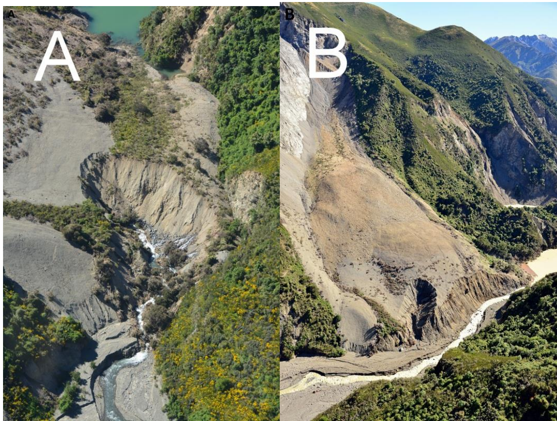
Figure 3: The greywacke-derived landslide dam in the upper reaches of the Conway River in the Seaward Kaikoura Ranges. This large dam developed flows through the permeable material of the dam under normal flow conditions (Photo 3A: J. Mitchell, 22/11/2016). On the 6 April 2017, 100-150 mm of rain fell in 24-hours and as a consequence this dam overtopped and breached, removing the landslide barrier and potential hazard. (Photo 3B: D. Townsend, 7/4/2017).
