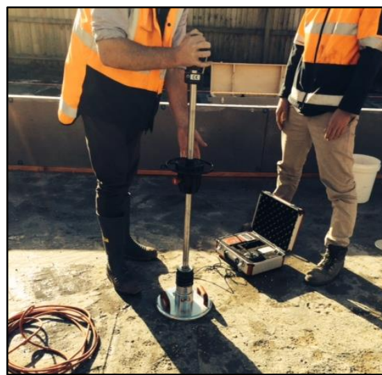
Figure 2: LWD equipment in use on PIC Raft shallow ground improvement
