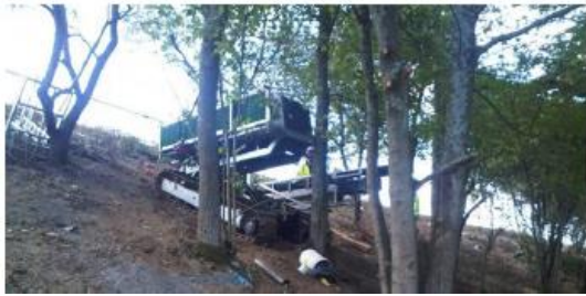
(a) self-climbing rig to install electrodes
