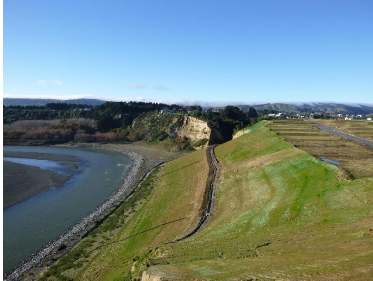
Figure 9: Photograph of completed realignment and cliff stabilisation works
