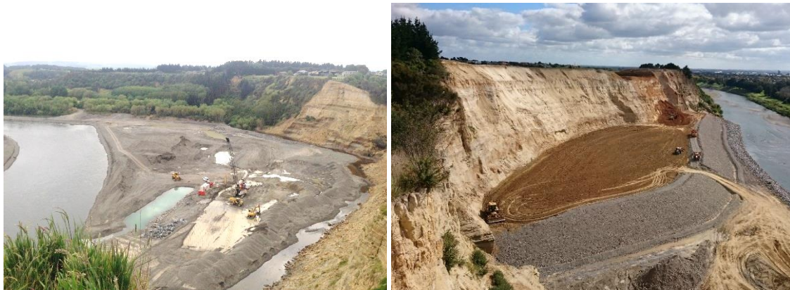
Figure 6: Looking south towards stone column installation, (9 December 2014)
