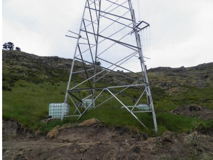
Figure 1: Transmission pylon prior to works
