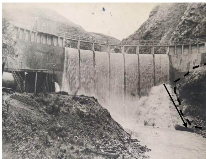
Figure 4a: Historical photo of No.2 Dam, showing potential slide block, arrow indicates foliation plane and dashed line indicates potential block of instability (date unknown).
