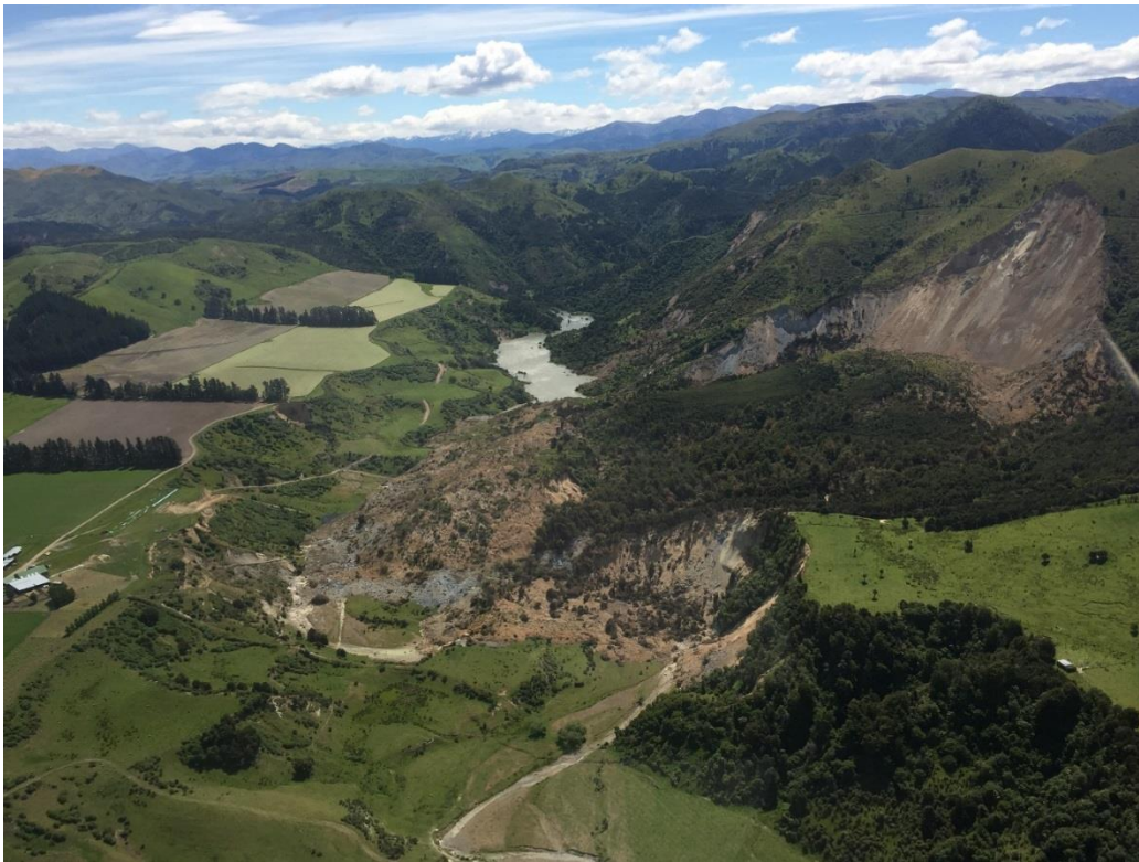
Figure 2: Landslide dam on the Leader River shortly after the earthquake. The landslide is a slump/block slide in a siltstone and is typical of the large landslides in weak Neogene rocks. The dam overtopped and partially breached in February 2017 (Photo credit: Environment Canterbury).
