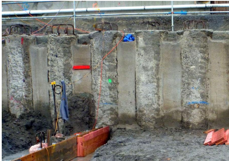
Figure 5. Hard and soft piles following basement excavation
