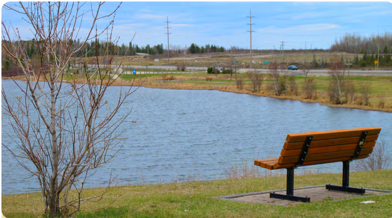
Stop 5: View across Gillies Lake and Highway 655 to a reclaimed tailings area that has filled the northeastern extension of Gillies Lake.
