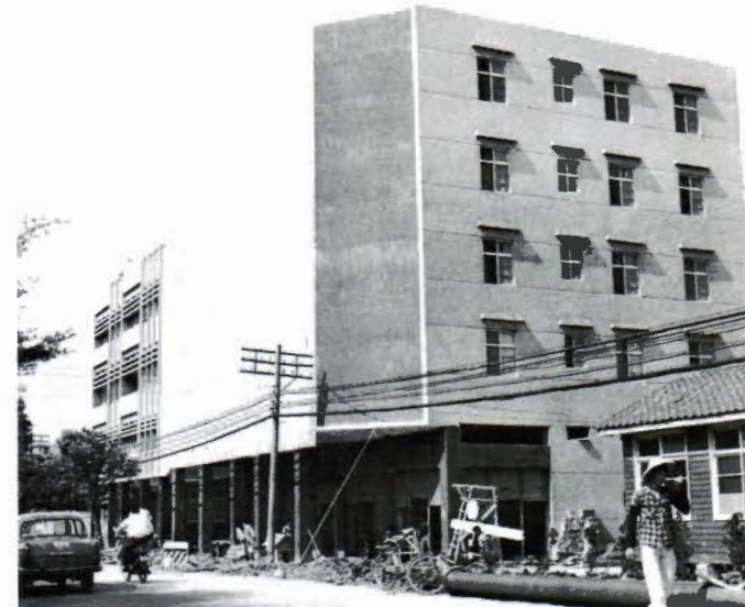
The Bahá'í Ḥaẓíratu'l-Quds at Taipei, Taiwan, R.O.C. Center is on third floor of this modern five-story building on one of the main thoroughfares of the city.
