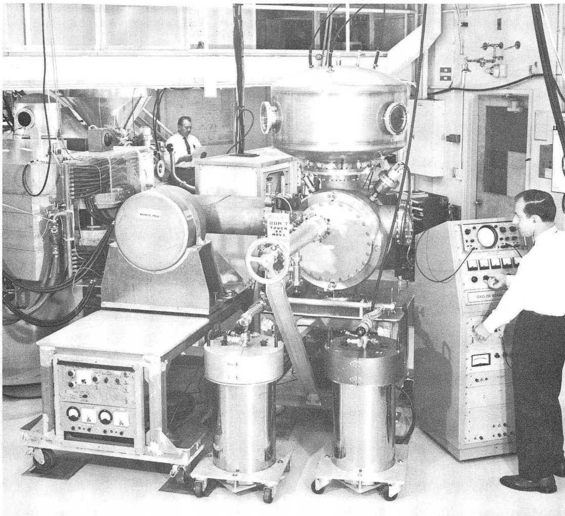
Fig. 2. View of cascade isotope separator from first-stage collector area.
