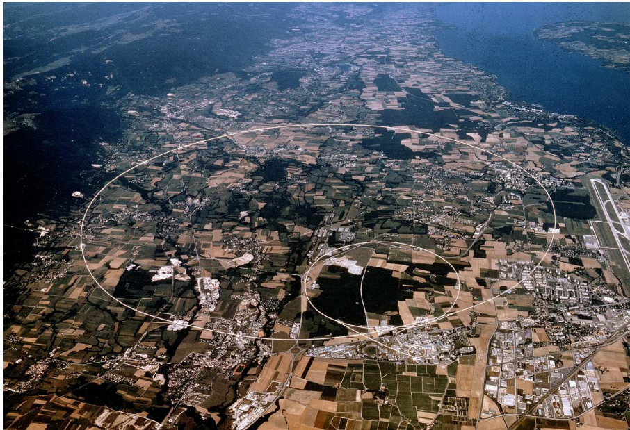
Figure 3.1: Aerial photograph of CERN. Accelerator rings are indicated by white circles [Cer91].
