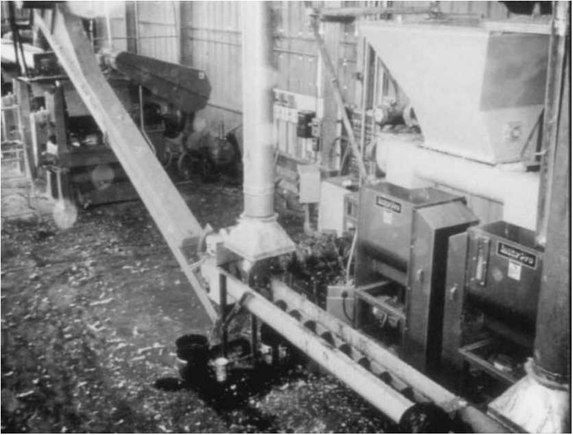
Figure 8. Photograph inside a modern extruding-expelling plant processing soybeans. (This figure is available in full color at http://www.mrw.interscience.wiley.com/biofp. )
