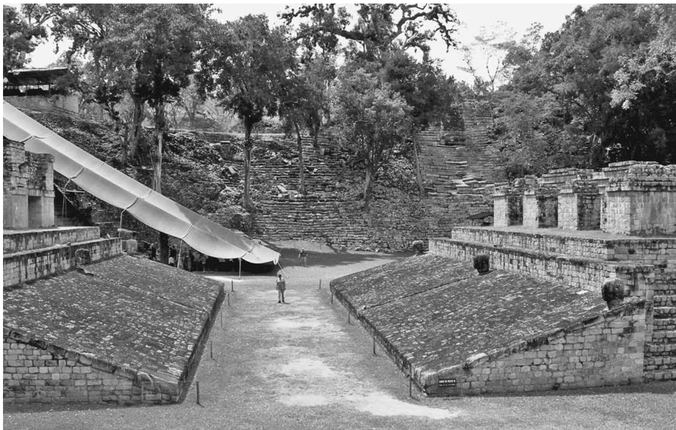
Final phase of Copán's ball court as commissioned by the city's ruler, Waxaklajuun Ub'aah K'awiil, in 738 C.E., looking south. The tarpaulin in the background protects the famous hieroglyphic stairway, the longest stone carved inscription in the entire Maya realm. (Courtesy of Janice Van Cleve)
