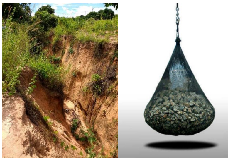
Figure 4-2 V-shaped gully and Rock Bag (source: Sumitomo)
