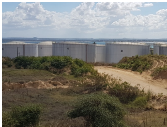
Damaged infrastructure at Nacala port
