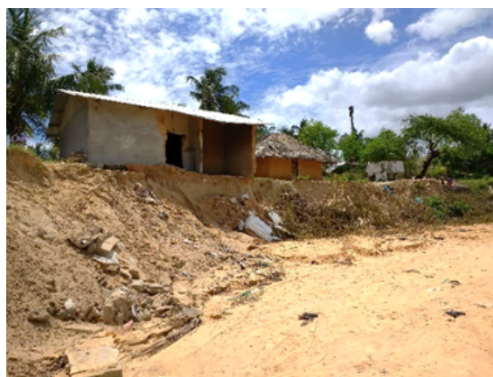
Destroyed house located at an erosion gully
