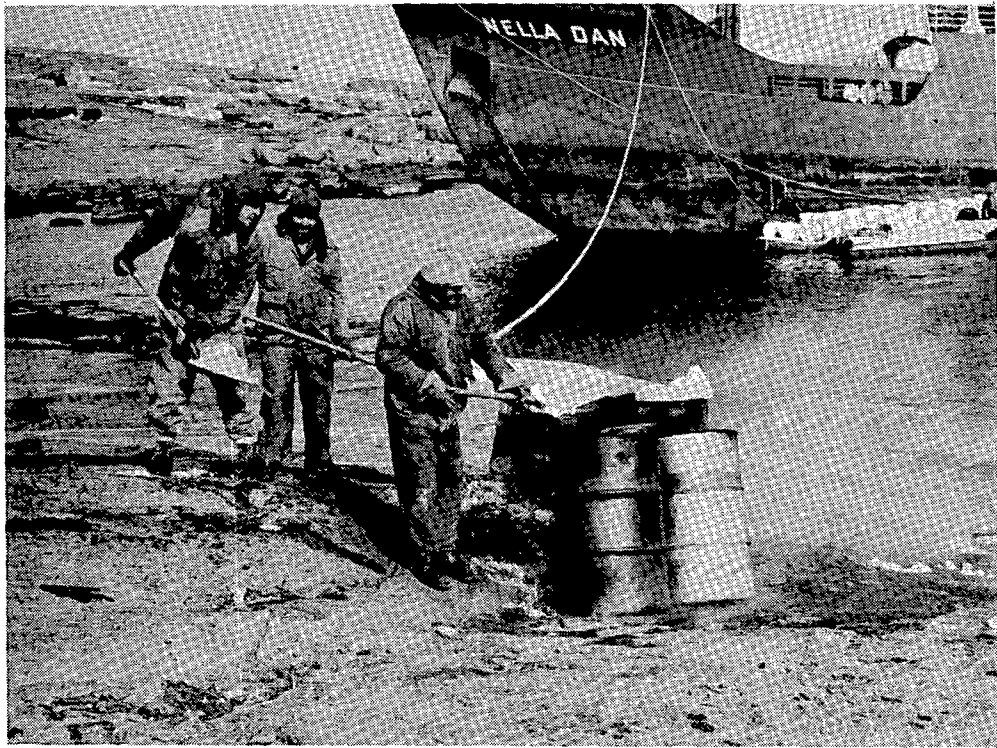
Fig. 1. Melting snow to produce heated mixing water for concreting. Drums are being heated by brown coal briquettes.
