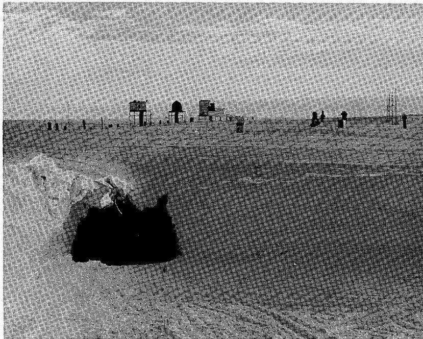
Fig. 2. Entrance ramp to Byrd Station as seen from surface.
