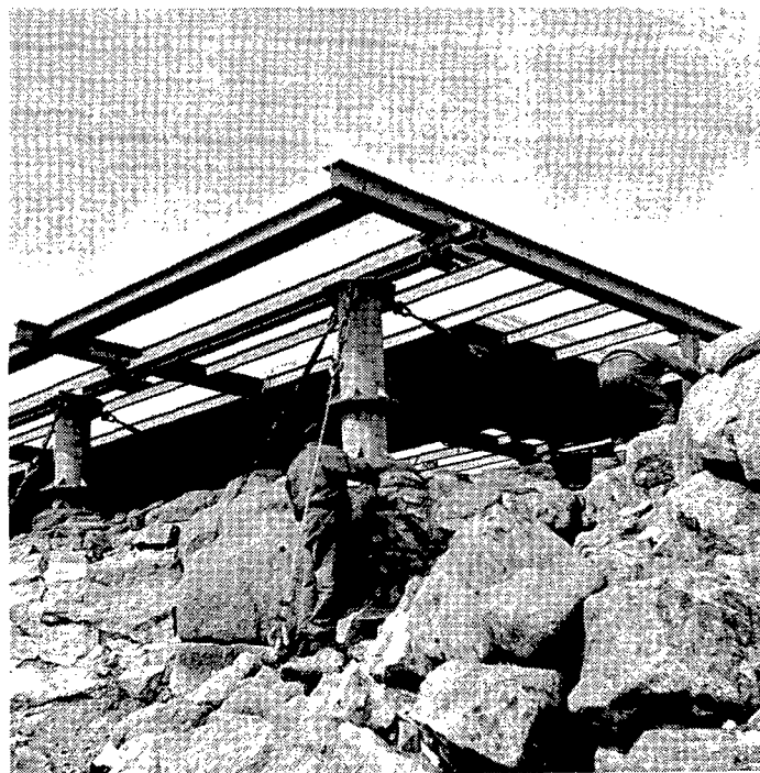
Photo 1. Construction of a metal platform. View of 2 posts with 2 components; the first with 1 m and 0.50 m components, the second with 1 m and 0.25 m components. 3 guy cables for each post. On the post; the templet. On the templet; the metal framework of the floor.
