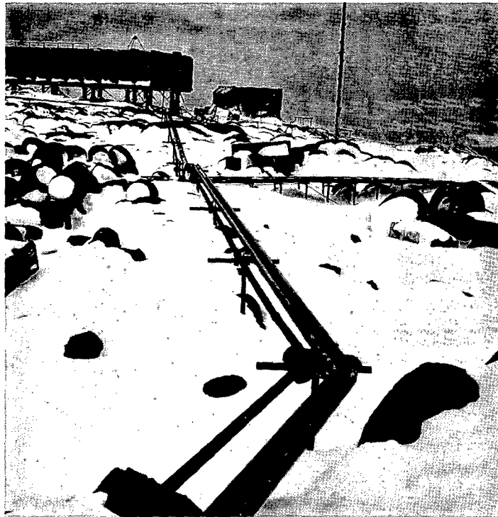
Fig. 26. Fuel-oil piping and electric cable-ways (1964). Set on tubular support to avoid being snowed up and iced.
