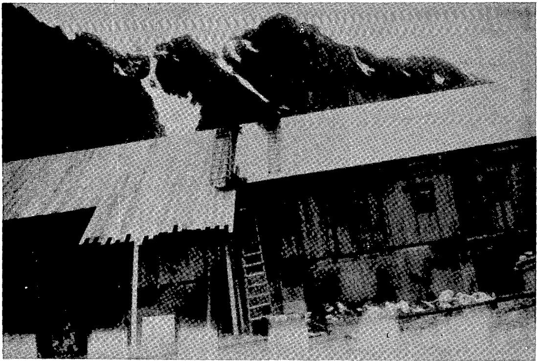
Construction of outer roof
