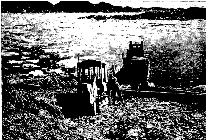
Winching Conex Boxes Ashore
