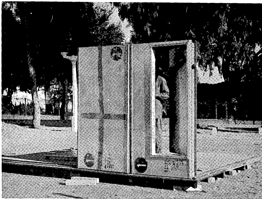
Placement of the first lateral boards
