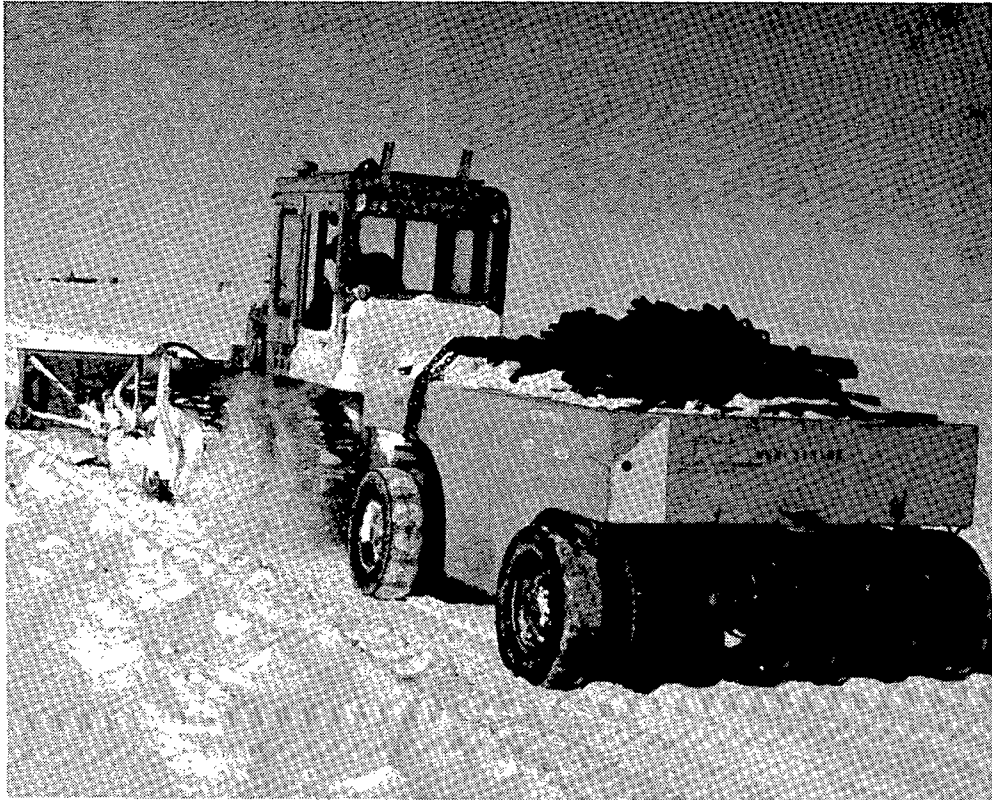
Fig. 6. Pneumatic-tired roller used to increase surface hardness of compacted snow roads.
