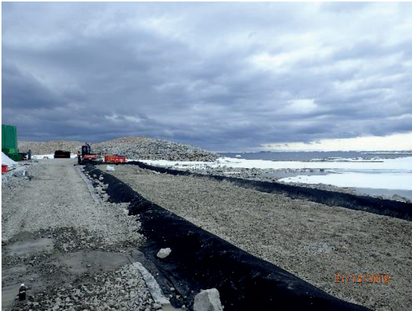
Photo 5: Protection layer of finer soil placed in biopile containment area.
