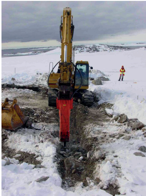
Photo 1: Digging trench for PRB wing in frozen ground.
