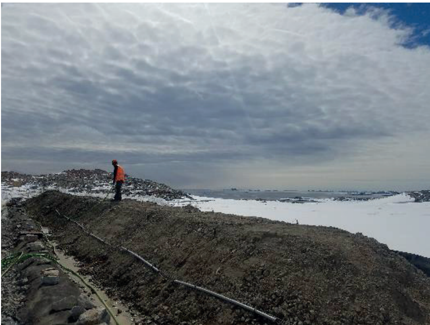
Photo 6: Manually circulating biopile leachate over soil during summer.
