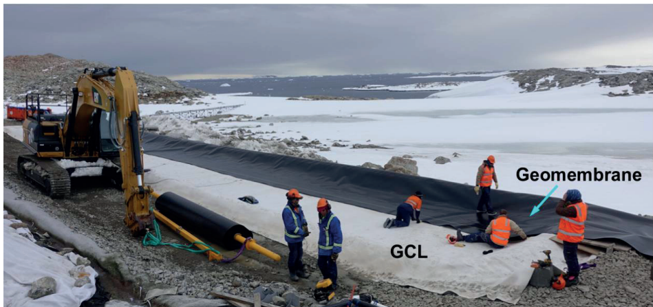
Photo 2: Installing GCL (white) and Geomembrane (black).
