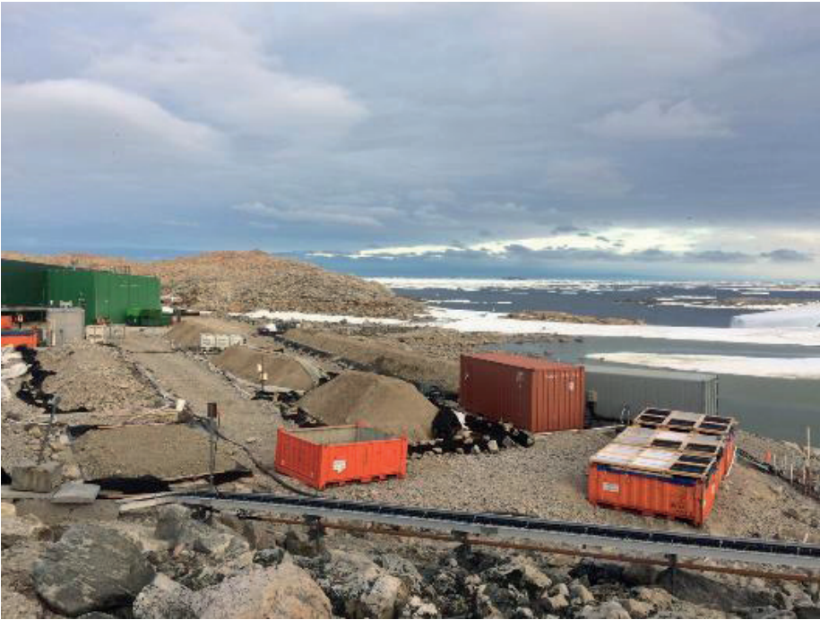
Photo 7: Showing multiple constructed biopiles in operation. Note uncovered for sampling purposes.
