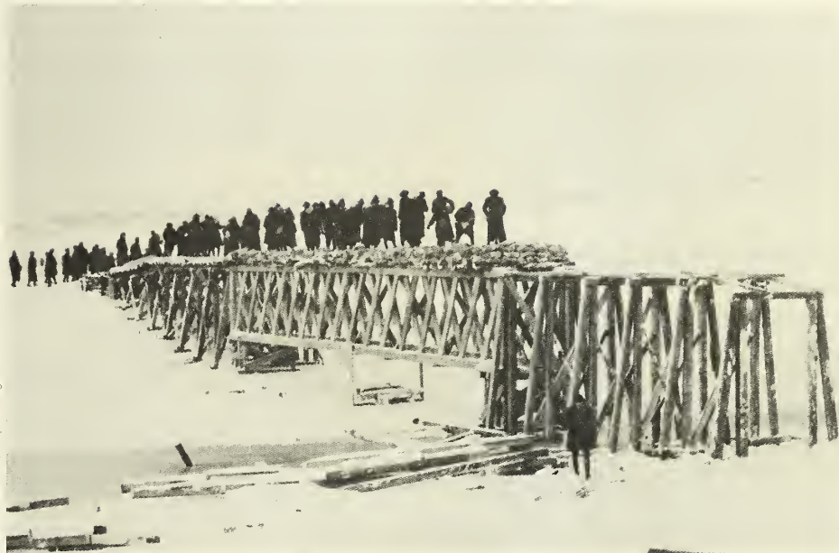
1st Engineers, 1st Division, test a bridge in Gondrecourt, France, January 1918.
