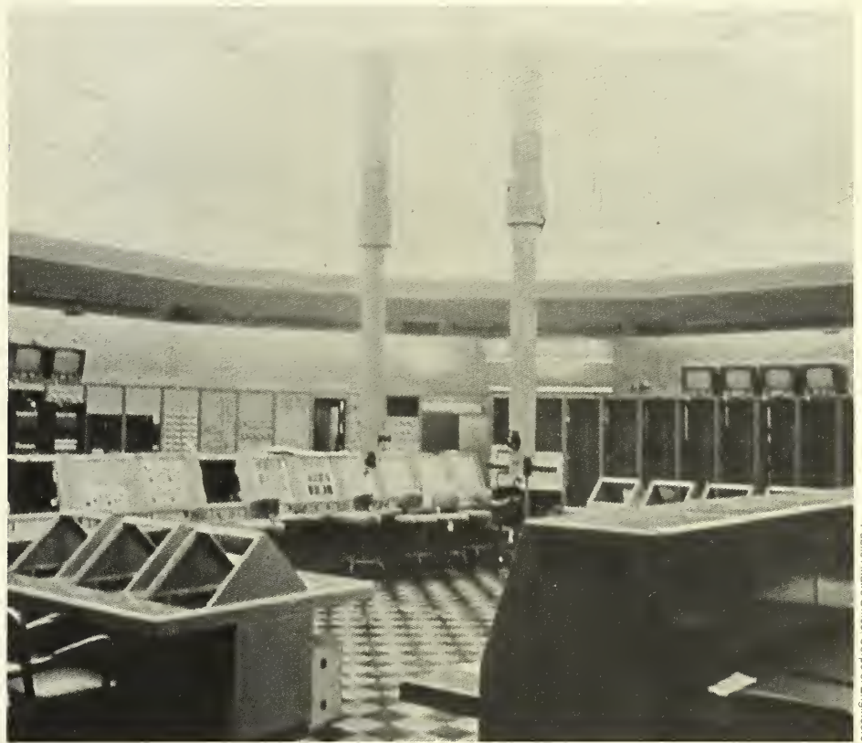
Pad 34 control room, Cape Kennedy.
