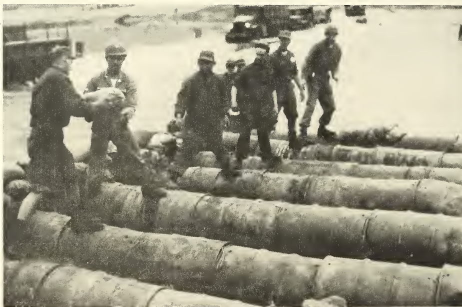
Building a "scrounge bridge" across the Pukhan River, April 1951.
