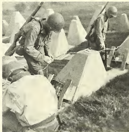
Placing explosive charges on concrete tank barriers along the Siegfried Line, October 1944.
