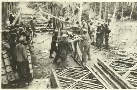
Working on a Bailey bridge over the Magampon River, Luzon, the Philippines, April 3, 1945.
