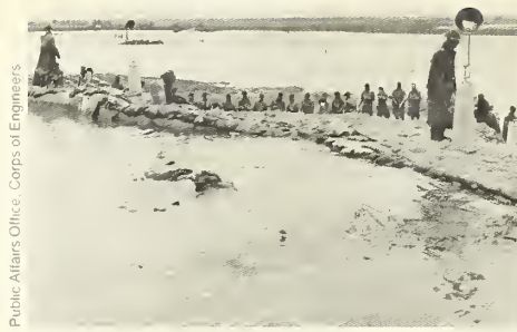
Carbide lamps illuminate sandbagging operations on Mississippi ring levee, 1944.
