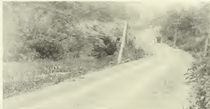
Looking east toward Cumberland, Maryland.
