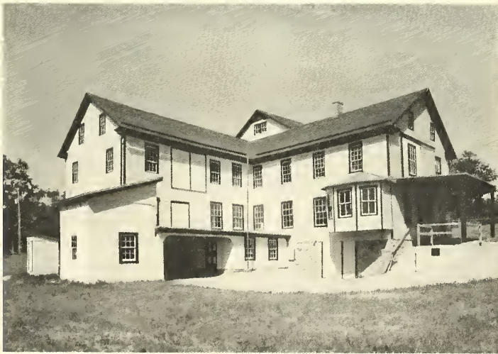
Restored Gruber Wagon Works, Bucks County, Pennsylvania.
