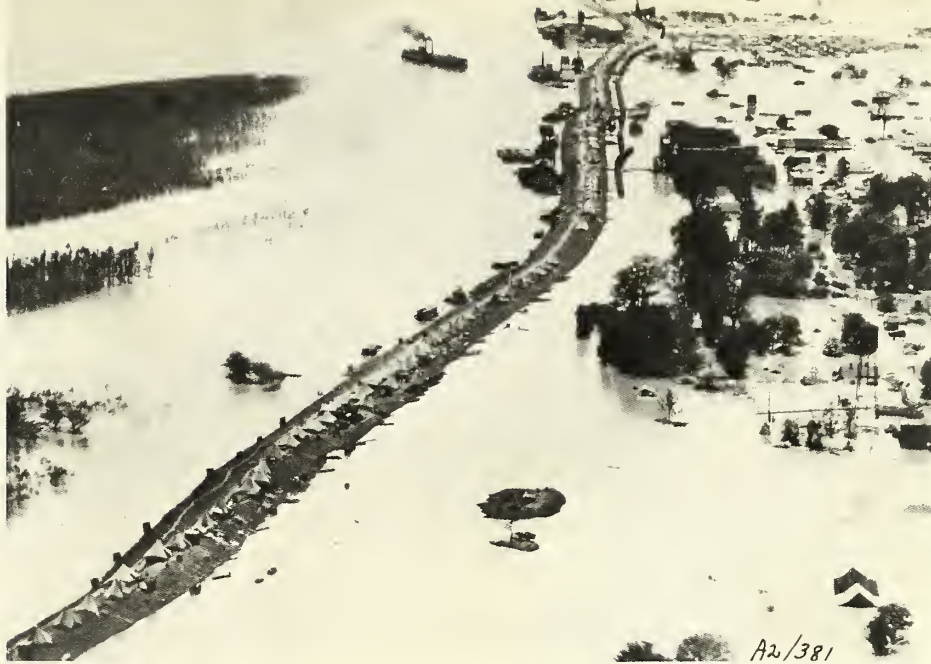
A2/381 Flood victims of Arkansas City, Arkansas, camp on a levee, 1927.
