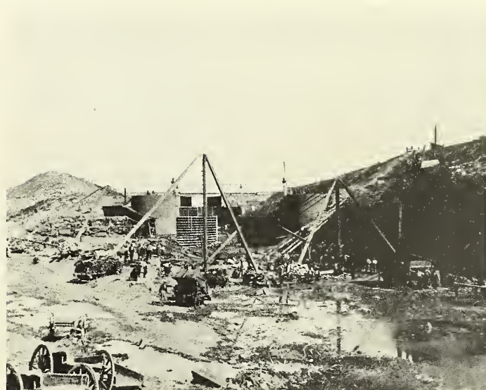
Louisville and Portland Canal under construction, 1871.
