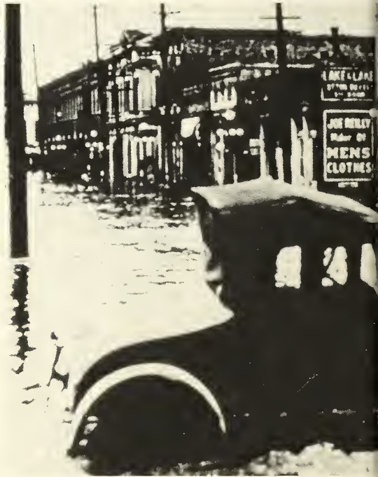
Flood at Greenville, Mississippi, 1927.
