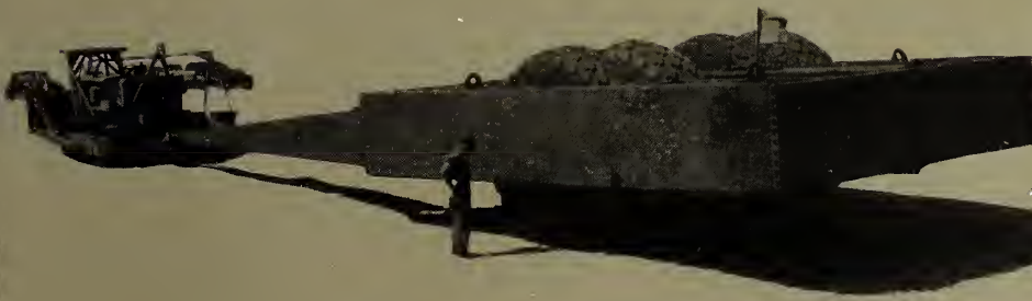
Historical Division, Corps of Engineers
