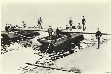
Students at Willets Point building a ponton bridge, 1889.
