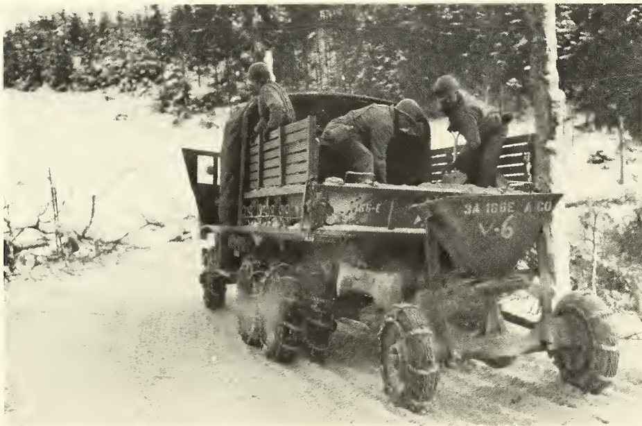
Members of 166th Engineers, sanding a highway with mechanical spreader. Near Wiltz, Luxembourg—1945.
