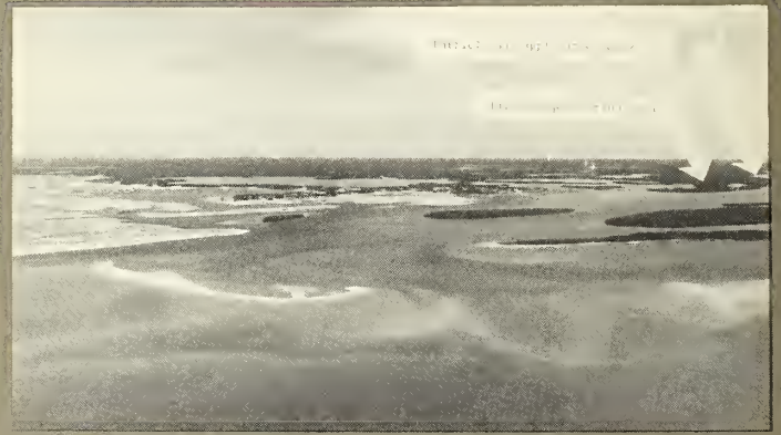
Historical Division, Corps of Engineers
