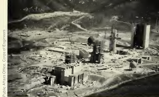
Space shuttle facility under construction, Vandenberg AFB, California.
