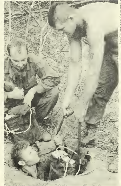
Engineer tunnel demolition team.
