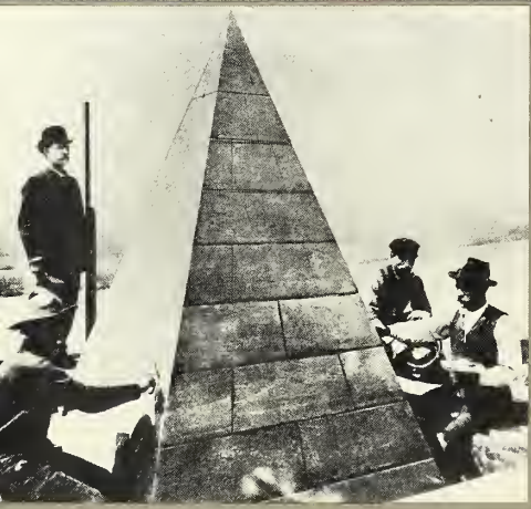
Workmen pointing tip of Washington Monument.
