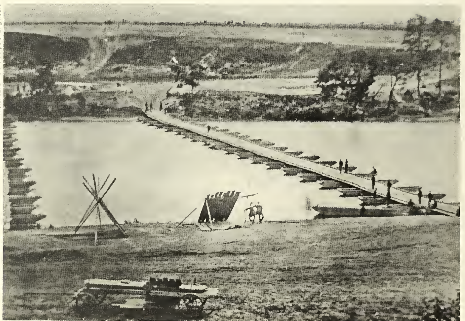
Ponton bridge across the Rappahannock River, built by the 50th and 15th New York Engineers, 1863.
