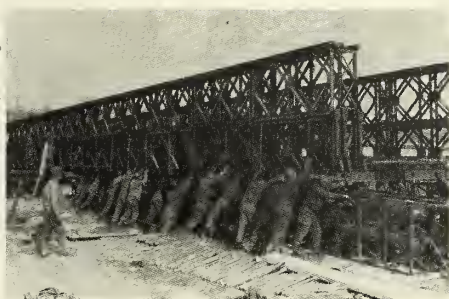
167th Engineer Combat Battalion, 1117th Engineer Group, builds the first Bailey bridge across the Rhine at Wesel, Germany, March 26, 1945.
