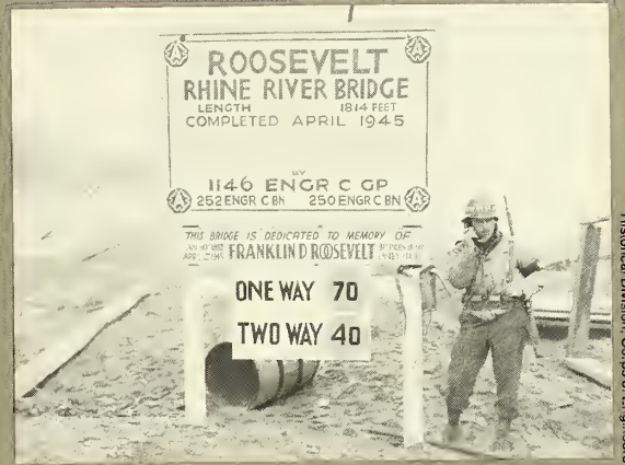
Historical Division, Corps of Engineers
