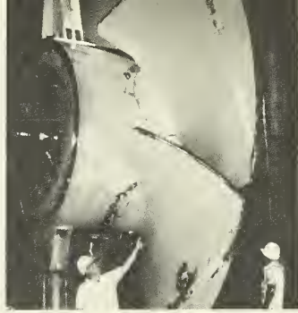
Power house turbine blade under repair.
