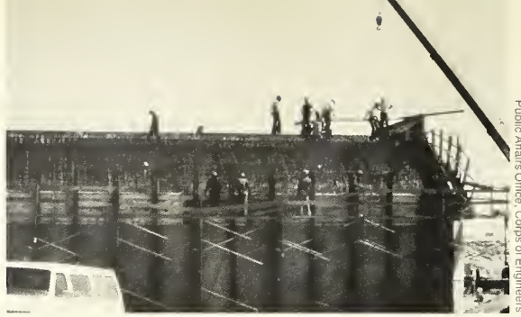
Israeli airbase under construction.
