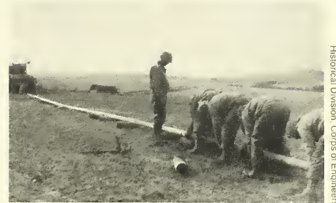
Connecting sections of 100-foot "snake" torpedo to pulling tank, Gorze, France.
