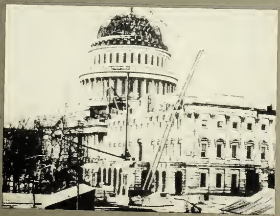
Historical Division, Corps of Engineers
