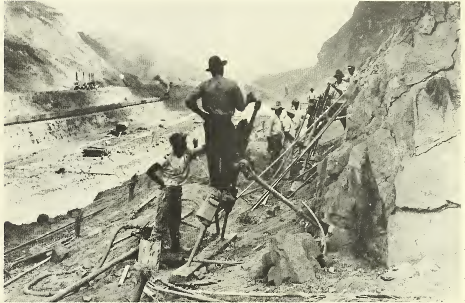
Drilling on Contractor's Hill at Culebra Cut, January 1912.
