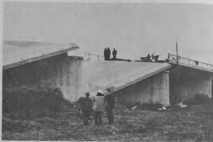
Pan-American Highway, Northern Chile section, earthquake of 8 July 1971
