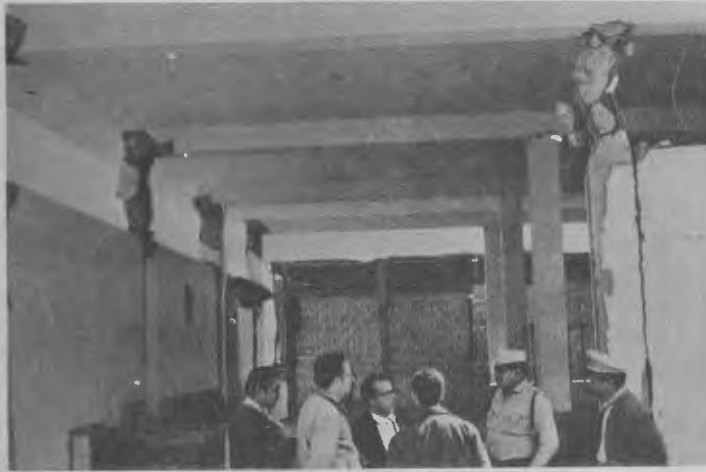
Huarney, Peru, earthquake of 31 May 1970
