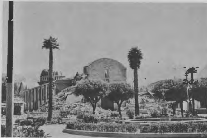
Huaraz, Peru, earthquake of 31 May 1970
