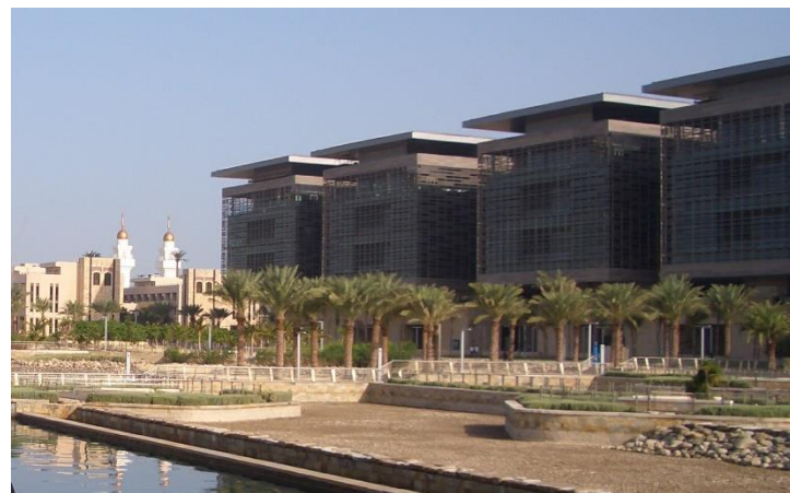
Figure 10. KAUST Laboratory buildings
