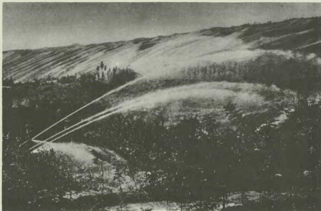
A sprinkler system fed by water from the Yellow River is used to accelerate the stabilization of shifting sand along the railway.
