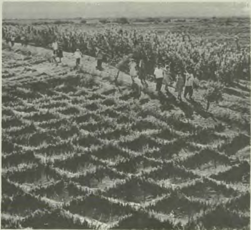
Construction of checkerboard protection to stabilize shifting sand near farmlands.
