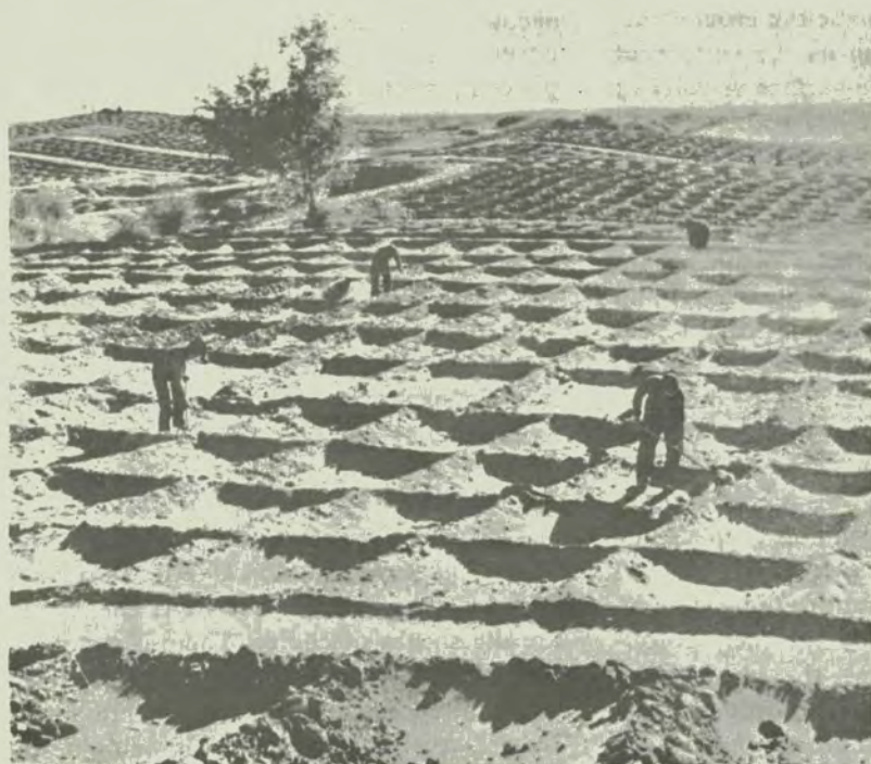
Clay deposits from the hollows between the sand dunes are successfully used to erect checkerboard protection.
