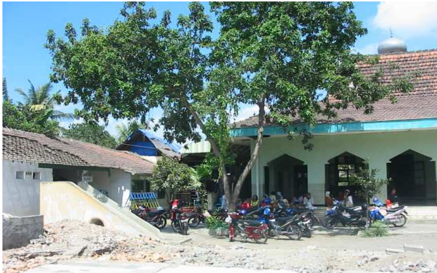
Photo of the collapsed buildings of TK ABA Ngangkruk and Bani Ibrahim's house, dated 19 October 2006
