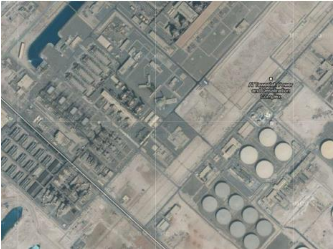
Figure 22: Key Target Examples: Gulf Desalination Plant
