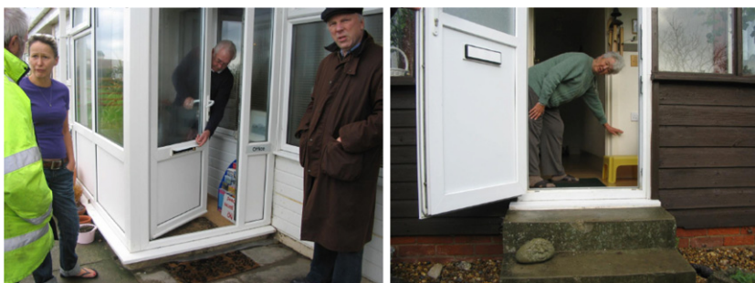
Figure 22 Photographs with Walcott residents indicating highest water mark during the event.
