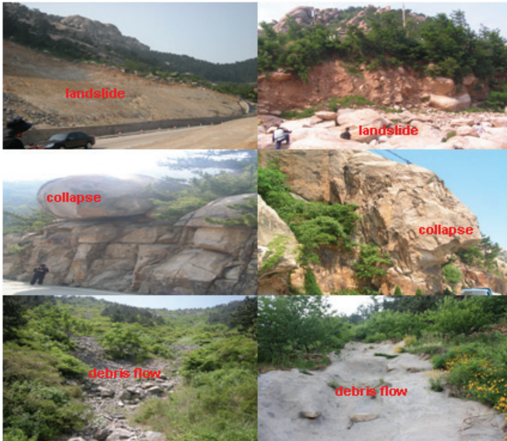
Fig.2 The photos of landslide, debris flows, unstable slope and collapse
