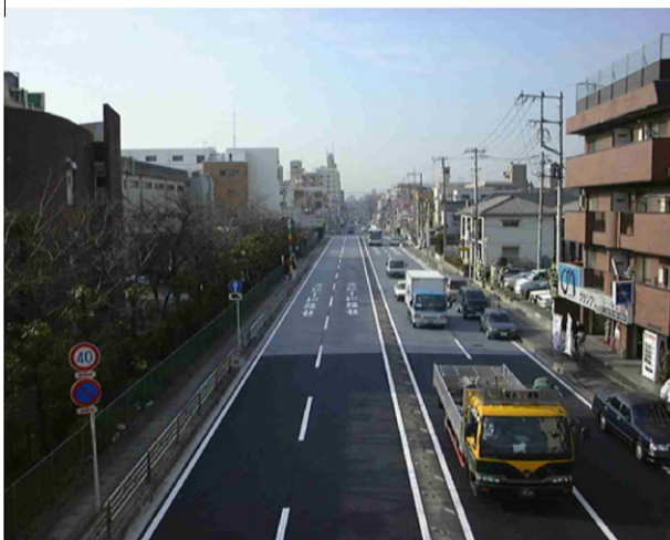
Fig. 12. Using TiO 2 photocatalytic material on roadway for pollution reduction: left – coating application; right – finished road showing a lighter color [36].
