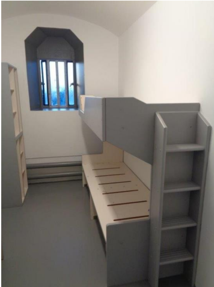
C wing cell after refurbishment
