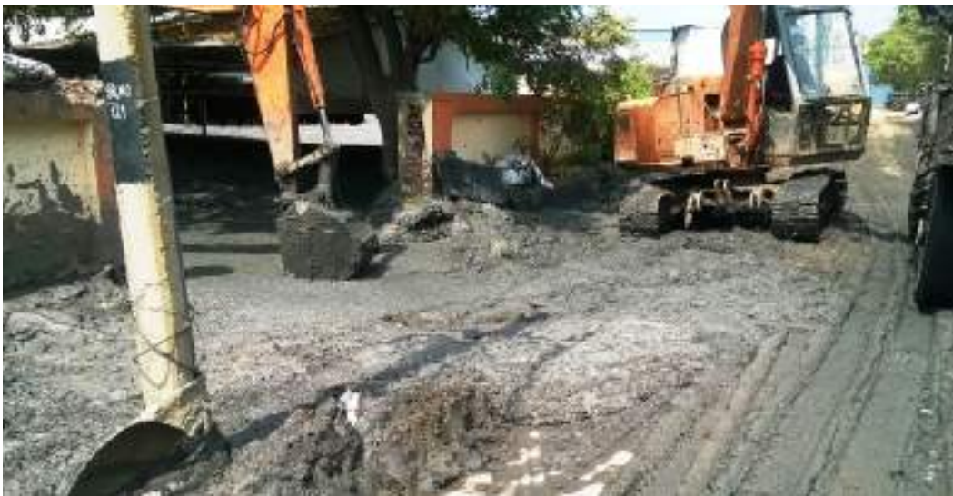
JCBs clearing the sludge-3rd day after the tragedy
