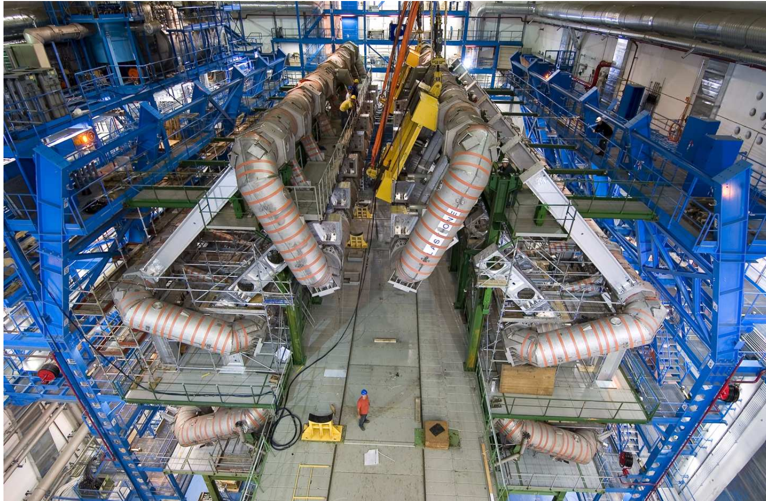
Installation of the 8th and final coil of the ATLAS barrel toroid
