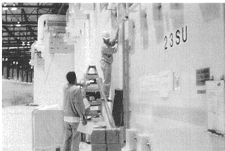
Figure 2.7.1: The periodical inspection of the limit switches of the optical hatch. (2001 July 11)
