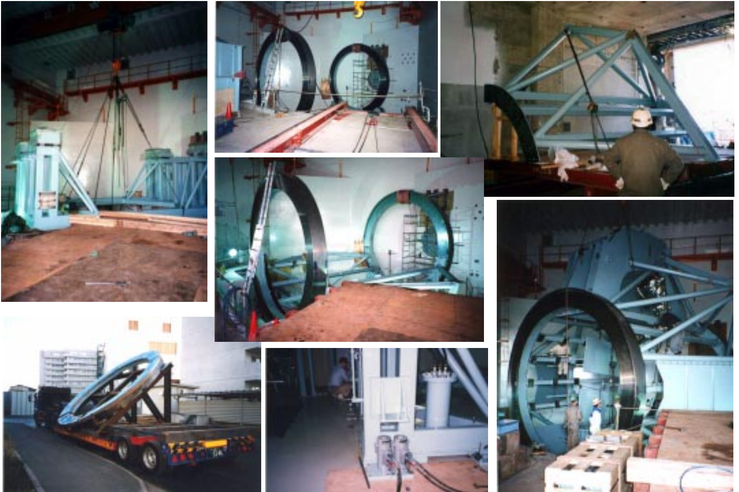
Figure 2-12: Images showing the assembly process of the isocentric proton gantry at the NCC. Source: Kataoka et al., 1999
