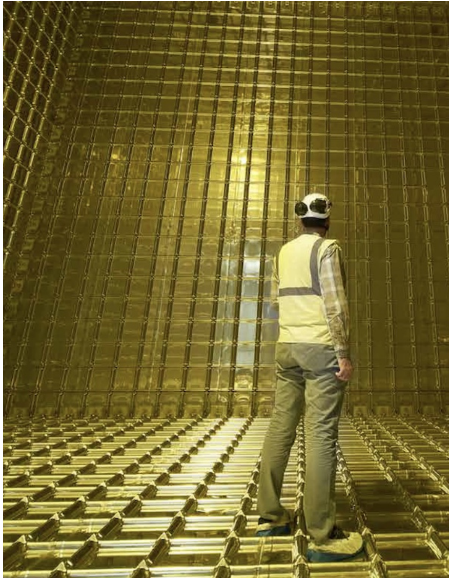
Figure 7.2: Interior view of one of the ProtoDUNE cryostats, before any detector components were installed, showing the membrane. The gold color is an artifact of the lighting that was set up to protect photo-sensitive detector components during installation.
