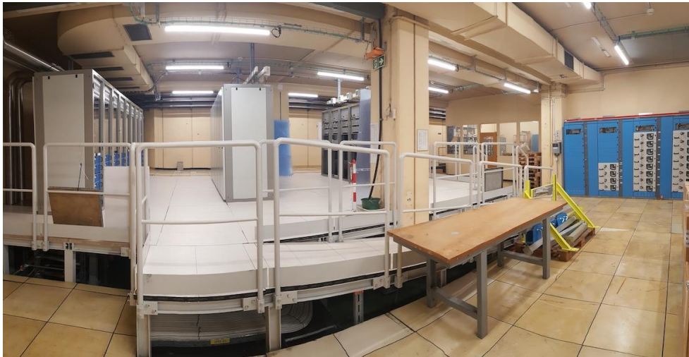
Figure 32. View of the renovated BRF1 equipment room.
