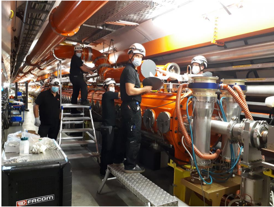
Figure 43. Connection of the RF line and FPC on a 200 MHz TWC.
