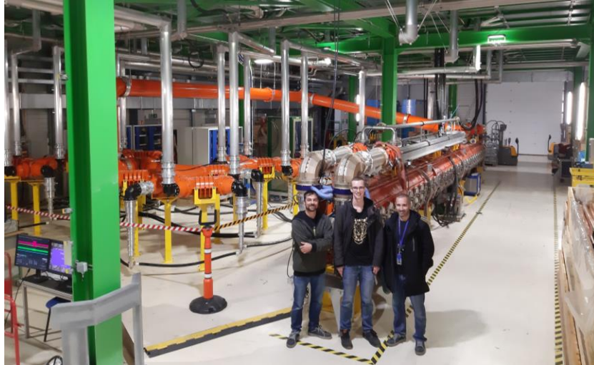
Figure 39. 3-dB-hybrids (left) and 3-section SPS TW accelerating structure (right) in BAF3.
