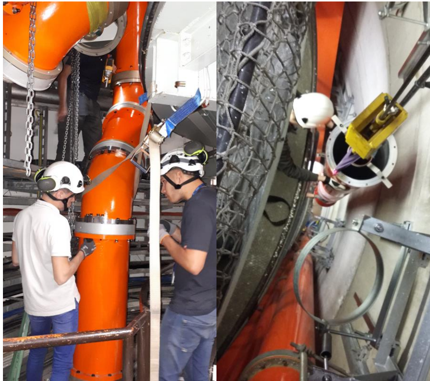
Figure 40. Installation of the coax line in TA3 tunnel.
