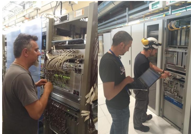
Figure 72. Both sides of the LN4-PSB trigger renovation.
