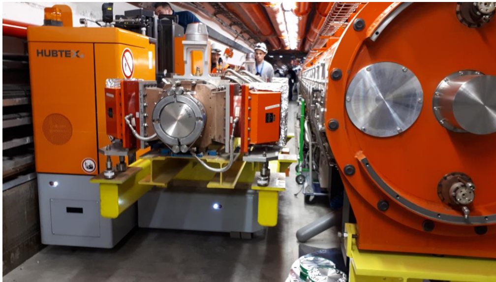
Figure 41. Transport of an 800 MHz cavity in LSS3.
