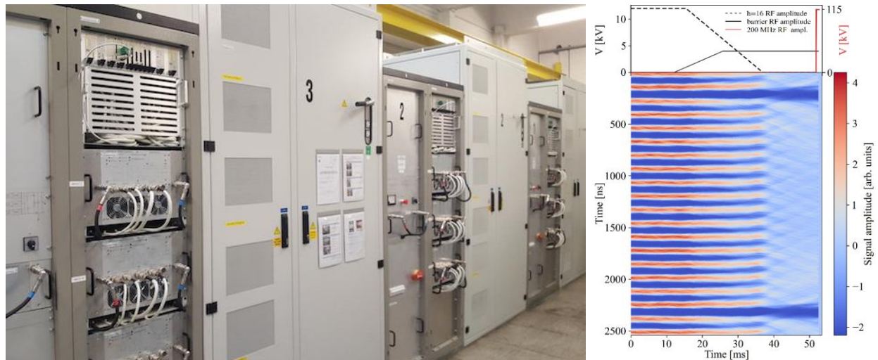
Figure 73: Left: New 24 kV power converters delivered by TE/EPC, feeding the final power amplifiers of the 40 MHz and 80 MHz RF systems in the PS; right: Measured evolution of the bunch profile from 16 bunches (0 ms) to one long bunch kept in a barrier bucket (50 ms).
