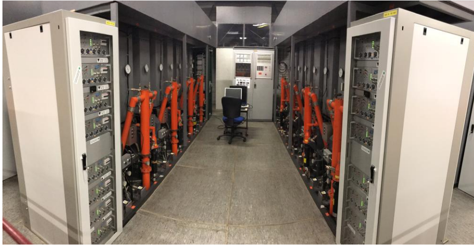
Figure 74: The new 1.25 kWp SSPA Driver amplifiers TTi Norte (Spain) in operation in the Philips 200 MHz system.
