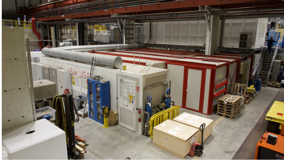
Figure 31 – Photograph of the laser hut in September 2019, after the new extension to the room. The first 2 m of the hut closer to the camera will be cut in spring of 2020 to accommodate a possible new experimental area requested by CERN. The equipment inside the hut must be moved before this.
