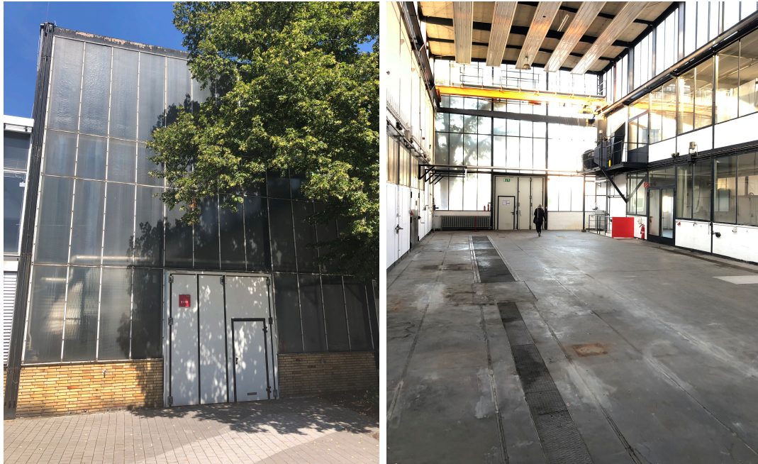
Figure 11.4: (Left) Facade of the temporary PUMA laboratory at TU Darmstadt. (Right) Inside of the laboratory. The laboratory will be equipped for 90 kW electric power grid and is equipped with a 3-ton crane.
