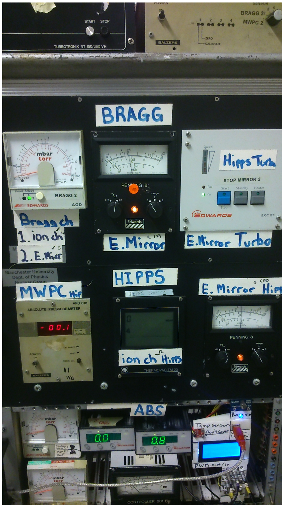
Figure 4.9: The vacuum gauge and controller cabinet to maintain and monitor the high vacuum environments within the STEFF detector, along with the non-vacuum gas detector regions.
