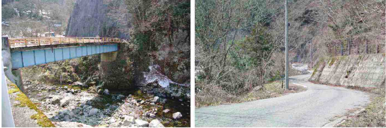
Figure 2.10: Photos of access road, and bridge. Shipment along this route must account for the 9-ton gross weight limit of the bridge and narrowness of the roadway.
