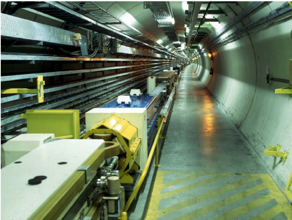
Figure I.2: The LEP tunnel.
