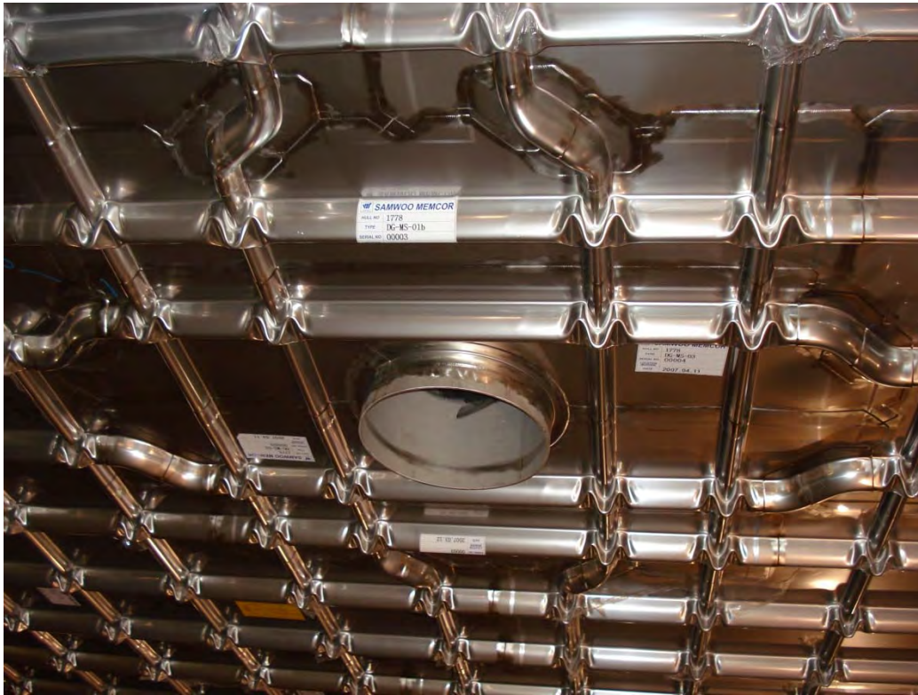
Figure 4-6: Nozzle in roof membrane cryostat (Figure courtesy GTT)
