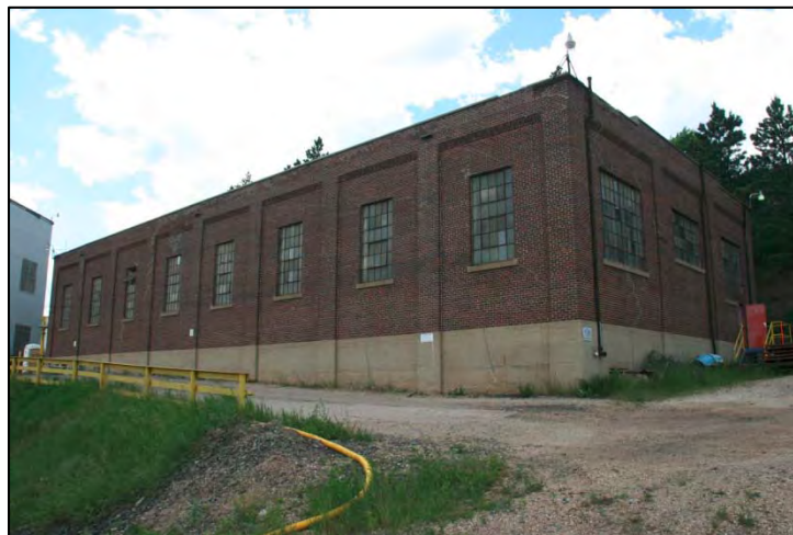
Figure 3-9: Photo of Ross Dry exterior (HDR)
