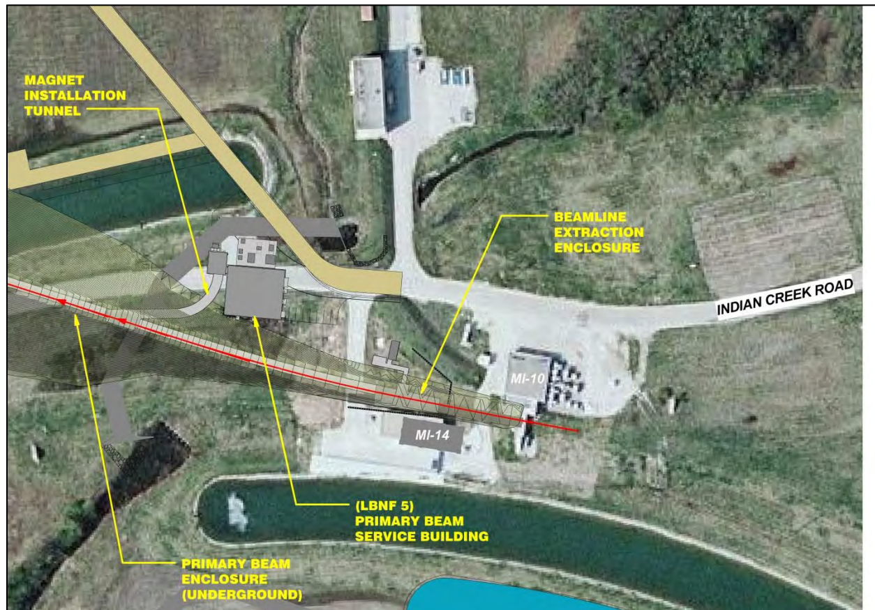
Figure 5-14: Beamline Extraction Enclosure and Primary Beam Enclosure – aerial view
