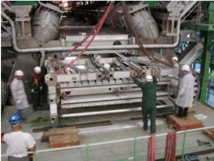
Figure 5.5: The sliding of a BML station in the Atlas apparatus.
