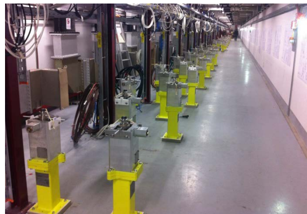
Figure 2 : Linac4 jacks ready for installation
