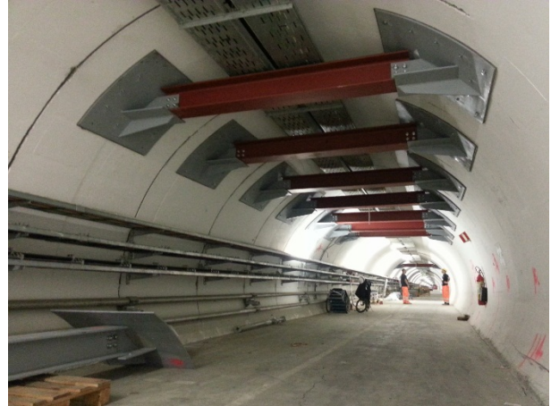
Figure 8: TT10 Tunnel reinforcements
