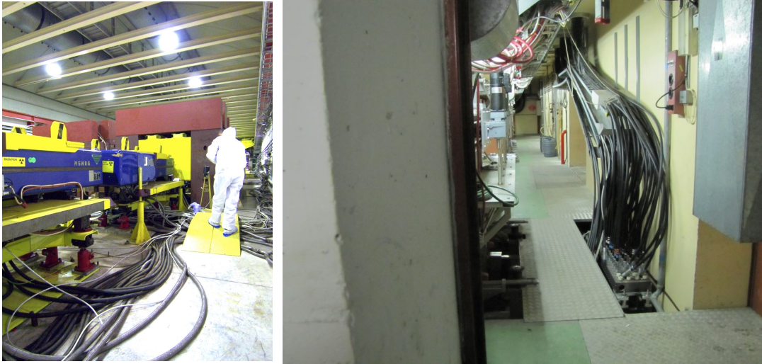
(a) A view of the SPS north area.
