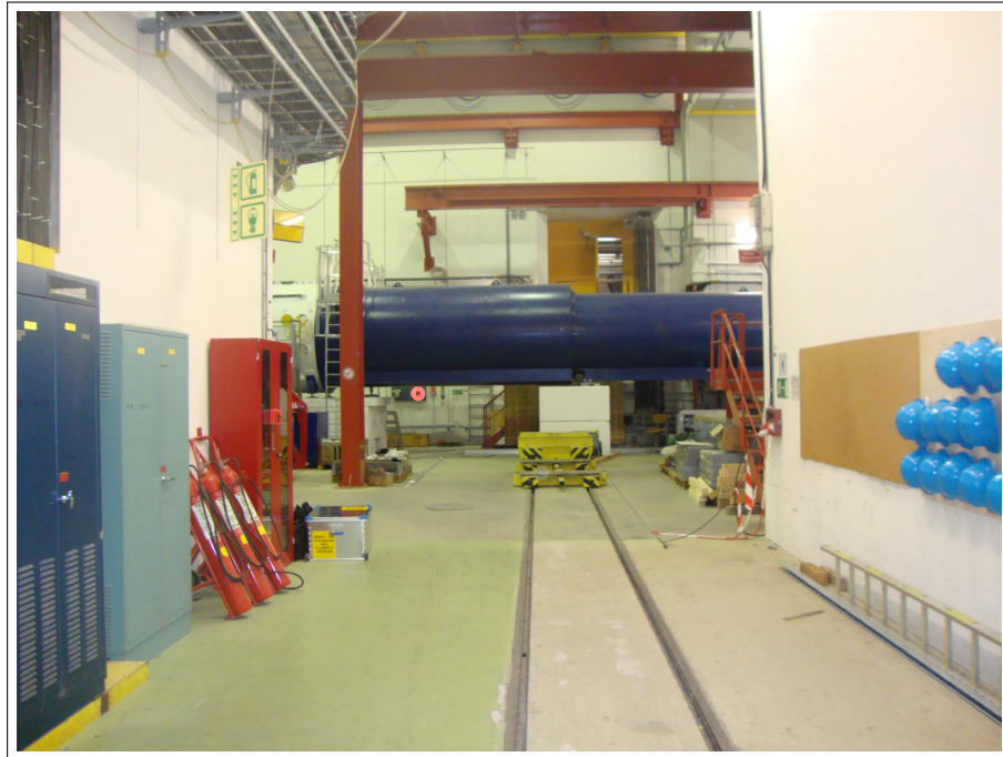
Figure 4.3: ECN3 tunnel area at CERN - view from the tunnel entrance.
