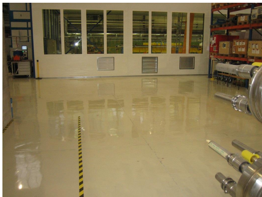
Fig. 8.4.2 – Cern Meyrin-site building 180.
