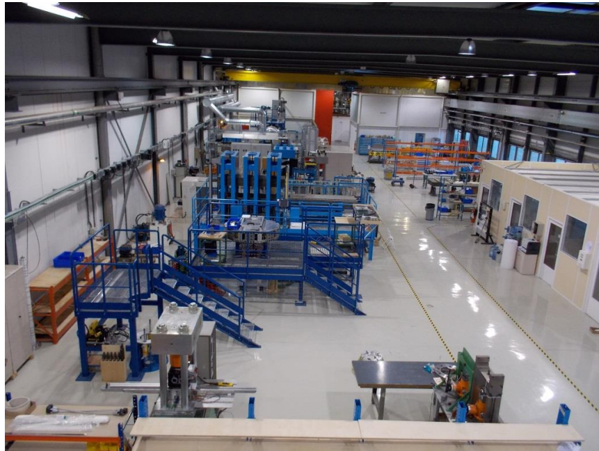
Fig. 8.4.1 – Cern Prévessin-site building 927.
