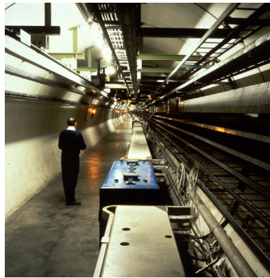
Figure 1.2. The LEP tunnel. A few magnets are visible on the picture.
