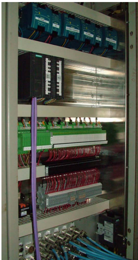
Fig. 3. Profibus DP: Remote IO
