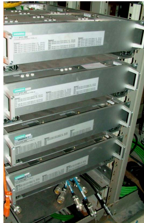
Fig. 4. Profibus PA: drawers of intelligent valve positioners
