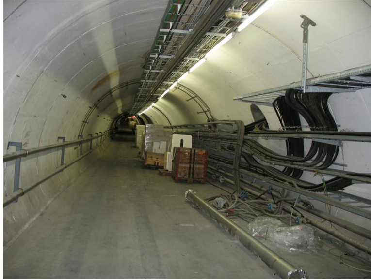
Figure 13: The TT61 tunnel at present.
