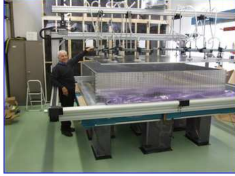
(b) Photograph of the module under construction to provide a sense of scale.
