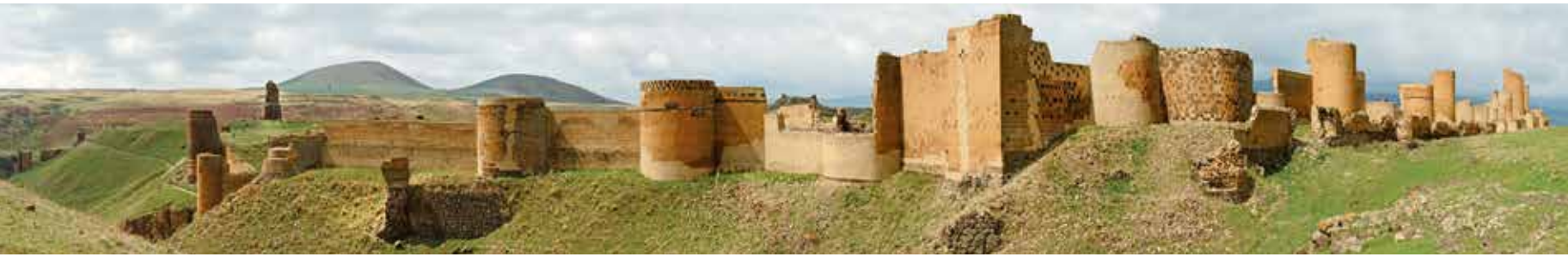
Fig. 21. Walls of King Smbat II at Ani, 10th–13th century with modern restorations
