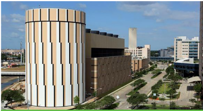
This 8.8-million-gallon chilled-water TES tank provides 75,000 ton-hours of cooling, integrated with 45 MW CHP at Texas Medical Center in Houston. 2 Photo courtesy of TECO
