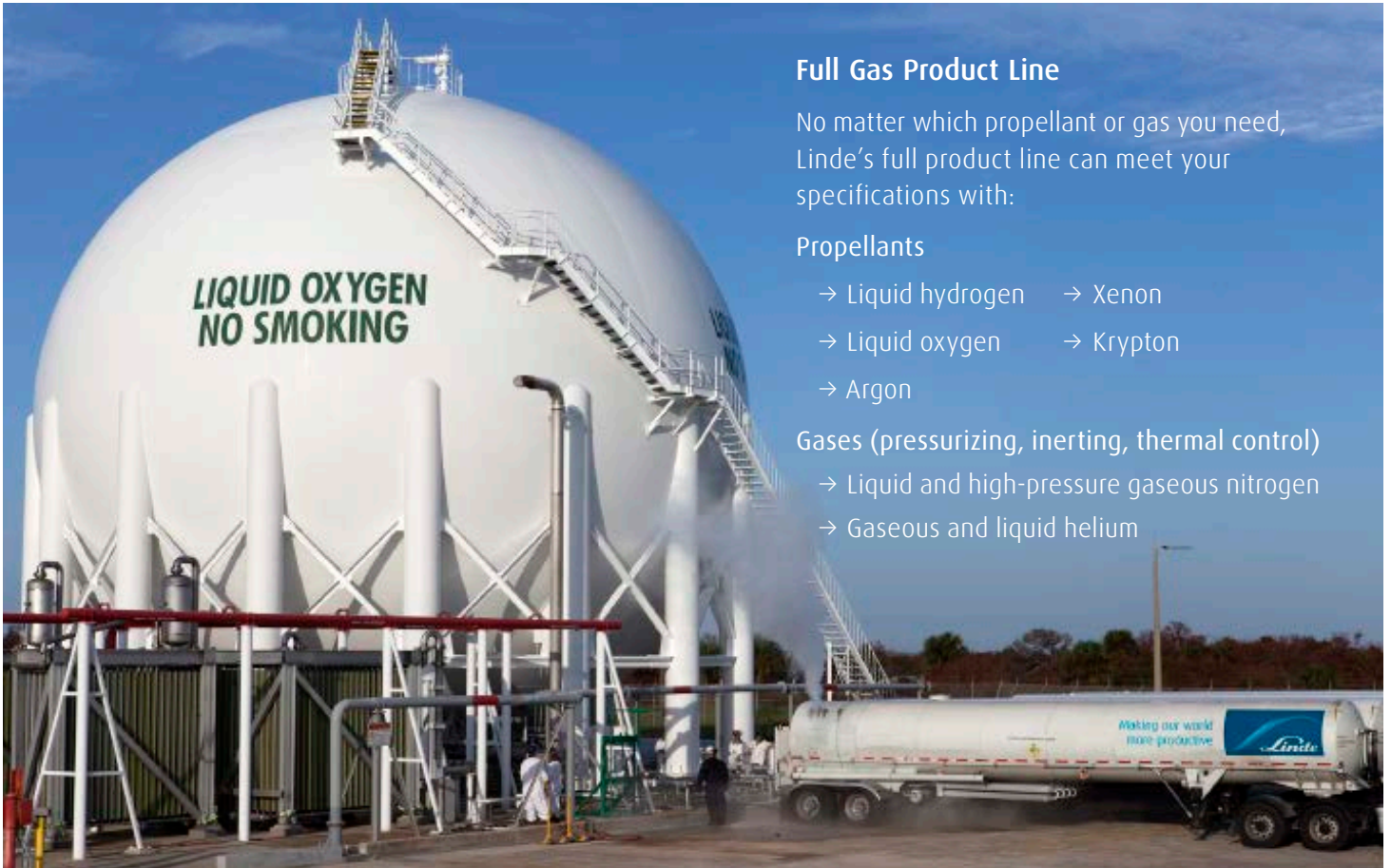
Linde delivery truck and liquid oxygen storage vessel at Kennedy Space Center pad 39B
