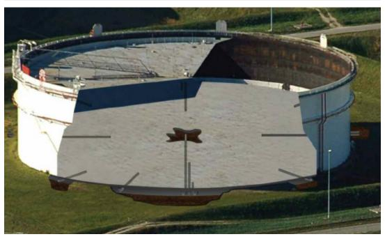
Tracer Tight leak detection is an industry recognized test method with precision sensitivity and compatibility with site operations. This method can locate leaks without any disruption of service, even in the largest of bulk storage tanks and the most complex of piping systems. Linde Services Inc. (Linde) provides Tracer Tight leak detection to a variety of facilities including but
