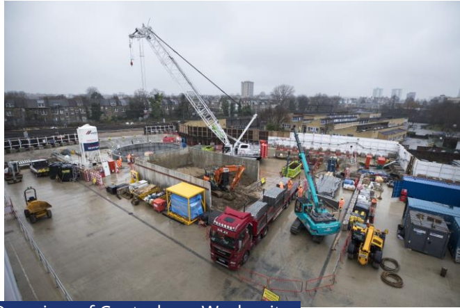
Overview of Canterbury Works site
