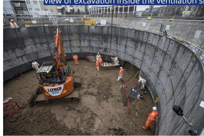
View of excavation inside the ventilation shaft
