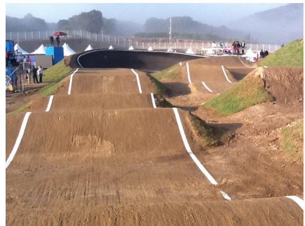
Jump footprint - the base is wider than the top. In this case, not enough space has been left for the access path between the straights.
