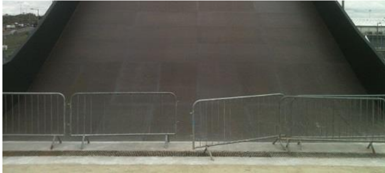
Drainage channel at the bottom of a start hill.
