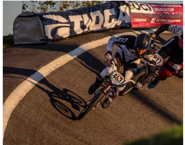
Example of a corner paved with asphalt. Notice how the pathway on top of the corner is also capped with asphalt. This stabilises the edge of the corner and prevents crumbling; it also keeps rain from penetrating behind the asphalt.
