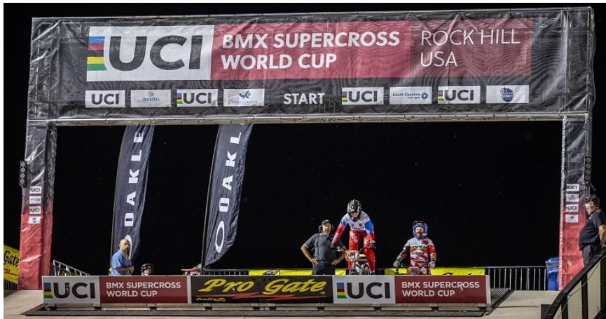
A well-designed start arch. This arch is bolted directly into the concrete pad that forms the top of the start hill.
