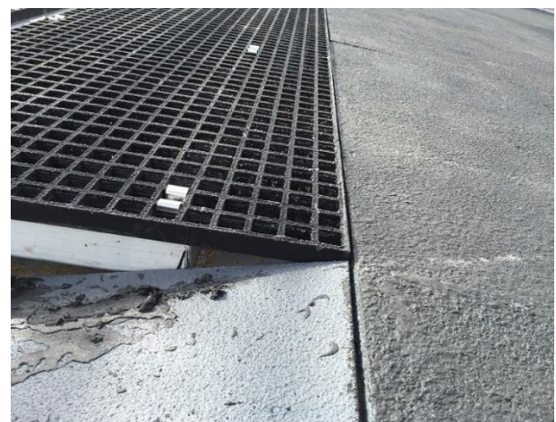
Gate Installation Best Practice - Gate platform slightly recessed to eliminate the small drop between the gate surface and start hill surface.
