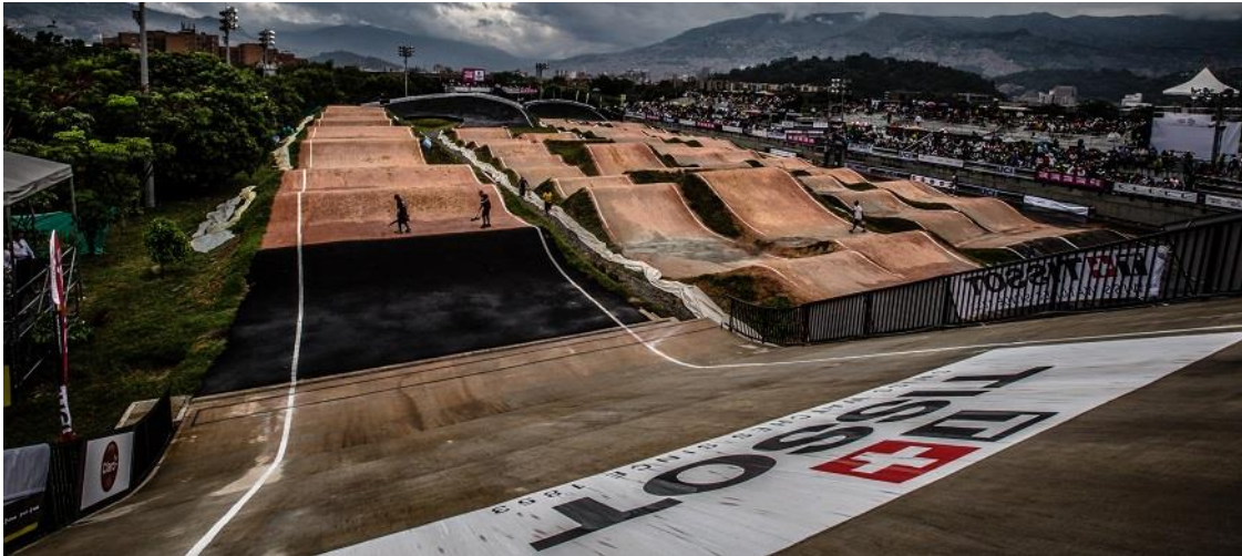
A start hill with a high grip surface. The high-grip decal extends the entire width of the start hill riding surface.
