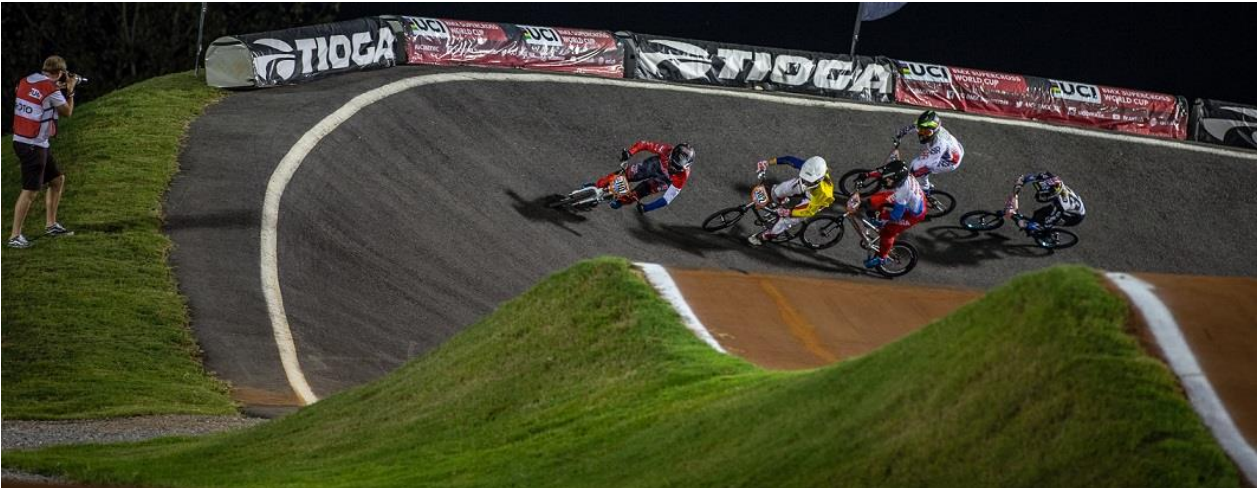
Gently sloped edges covered with grass prevent erosion, and reduce the risk of injury in case a rider is ejected from the track.
