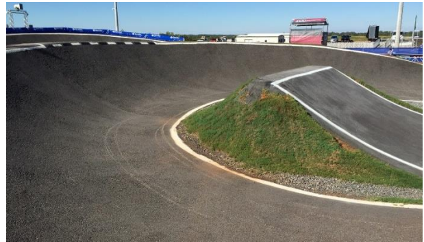
Berm jump with lines for visual reference.
