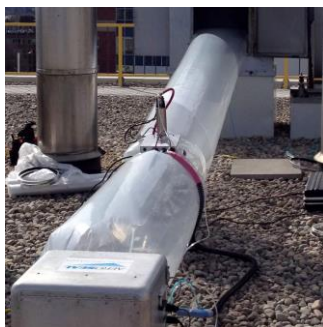
Figure 6: Sealed duct system connected to an Aeroseal aerosol sprayer and fan
